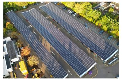
The 617 solar panels will reduce carbon emissions by 43.7 tonnes per year, saving the Trust £75,000 yearly. The electricity generated will cut the demand of grid electricity by 15%, enough to power 60 UK houses.
